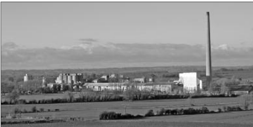
Westbury cement works, now under threat of demolition
