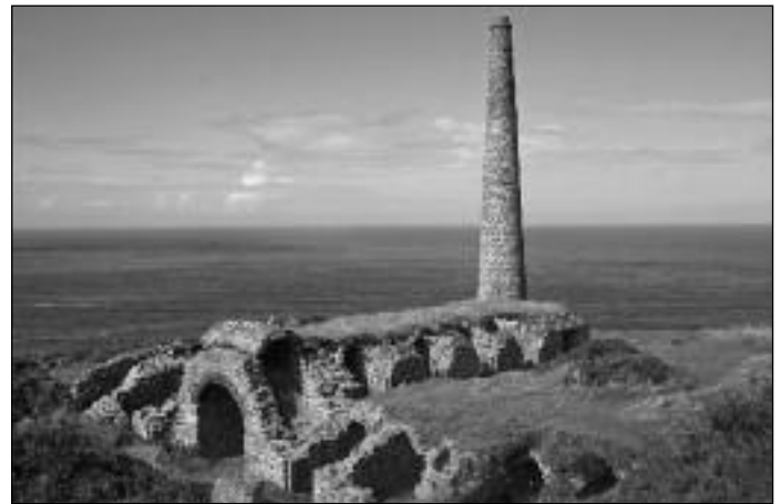
Arsenic calciner and flues at Botallack
