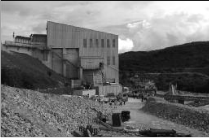
The Melbur dry processing china clay plant
