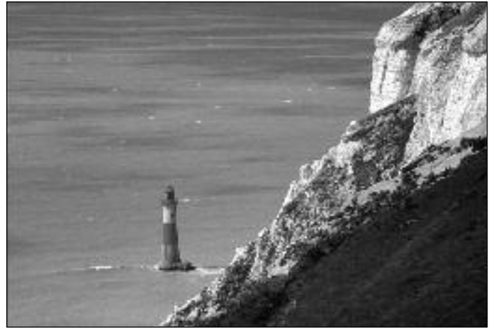
The lighthouse at the foot of the famous chalk cliff of Beachy Head may soon become redundant. The 1902 granite tower has been unmanned since 1983 Photo: Peter Stanier
