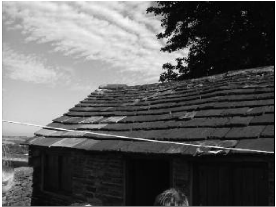
The stone roof of the Hoylandswaine nail makers workshop
