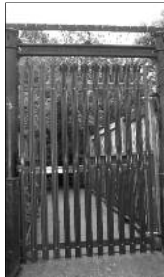
Original footbridge iron work bearing the name of Louis Harper at Grimsby Photo: Tim Mickleburgh
