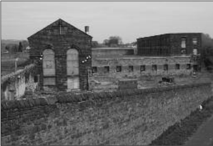
Pendle Street Shed, Nelson, Lancashire, is a fine example of a room-and-power weaving mill of 1885. It has already lost its chimney and boiler house, and now faces a threat of total demolition Photo: Roger Holden
