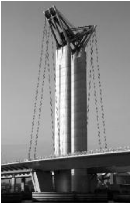
Rouen's modern lift bridge, the Pont Gustave Flaubert, is a distinctive landmark Photo: © Bill Barksfield 2010
