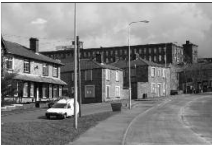
Brierfield Mill, a rare example of a cotton spinning mill in East Lancashire, proposed for conversion to an Islamic Girls Boarding School. Note the terraced housing which has been empty and boarded up for several years as a result of a misguided council 'regeneration' project Photo: Roger Holden
