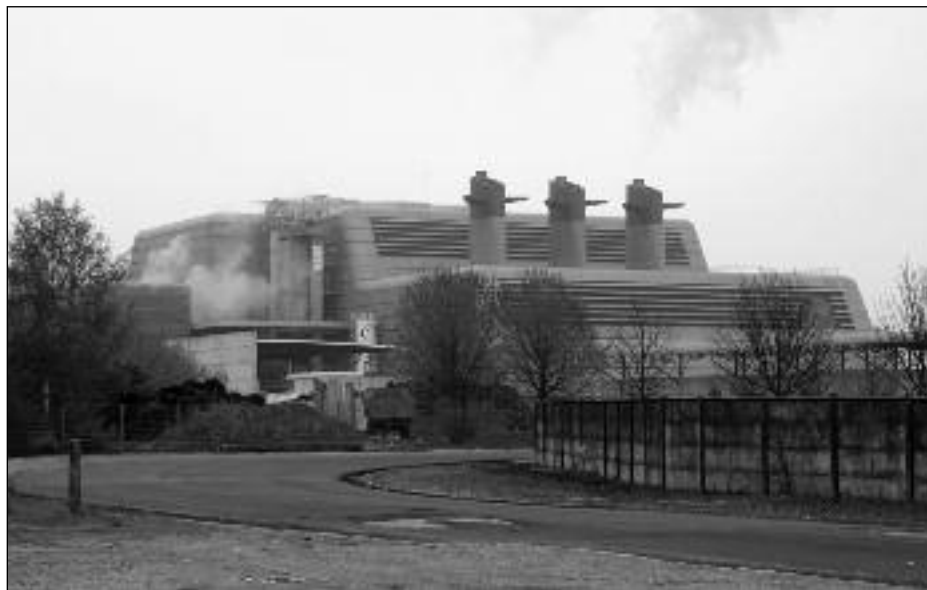
An ocean liner? The remarkable design of the waste incinerator and electricity generating station at Rouen
