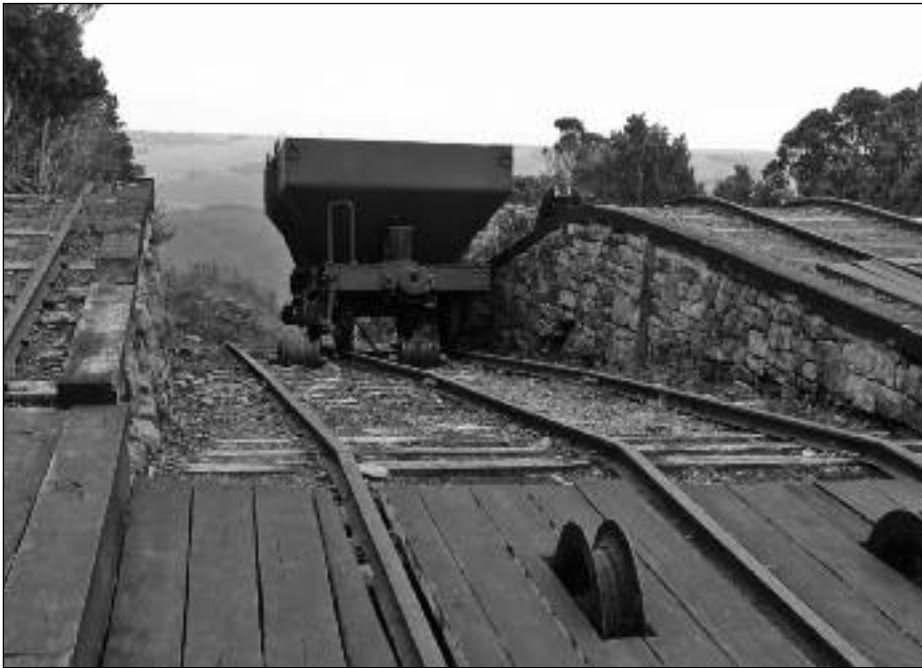
Denniston Incline top. Beyond the grassy hump to the left of the wagon the descent becomes vertiginous
