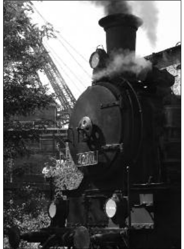
Michal Colliery and locomotive, Ostrava, Czech Republic
