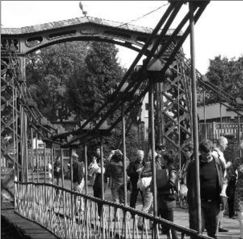
Suspension bridge of 1827 at Mala Pane ironworks, Ozimek, Poland
