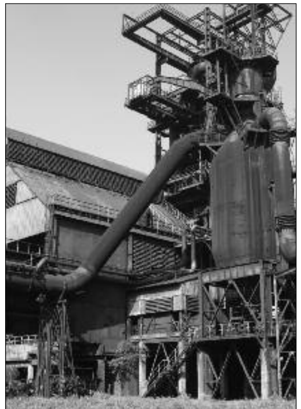
Blast Furnace No. 1, Vitkovice, Ostrava, Czech Republic
