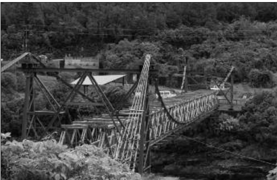
The bridge at the Brunner mine. Originally a combined road and railway bridge, it is now for foot passengers only
