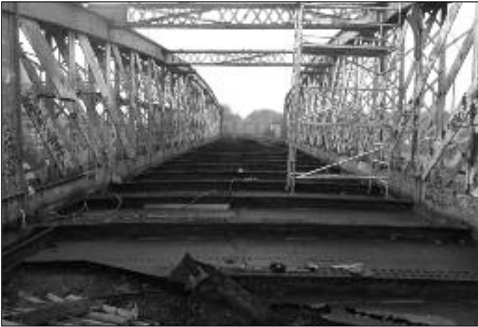
The ex-GCR Bowstring Bridge in Leicester under demolition
