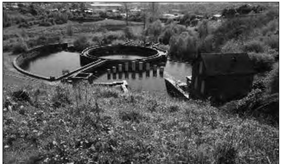
*The weir and flow measuring system below Bottoms Reservoir at Tintwistle*
