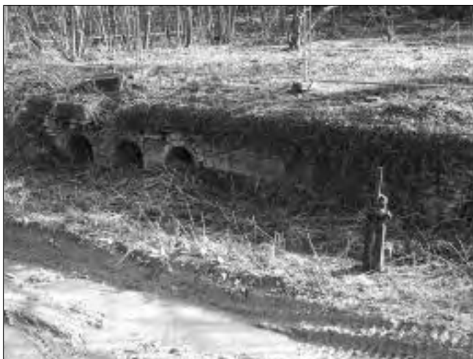
Exposed remains of the early nineteenth century Whitehouses pumping station. The arches are where water was pumped out into the Grand Union's Wendover Arm from the lower-level Wilstone Reservoir Photo: Henry Gunston
