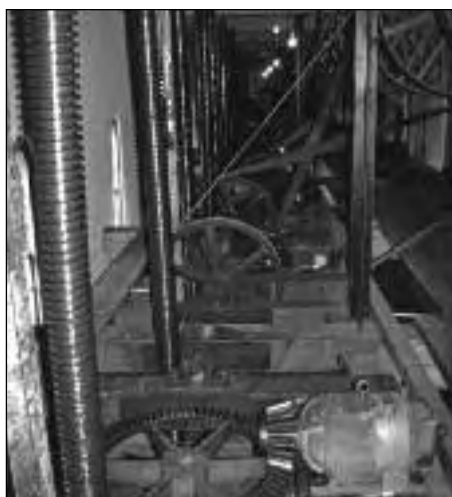
The line shafting and screws which raised the gates
