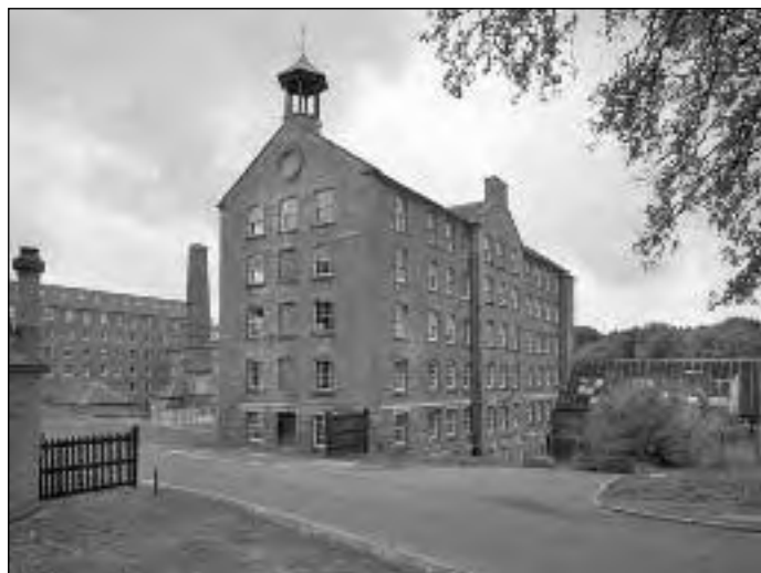
Bell Mill (1790), Stanley Mills, Perthshire
