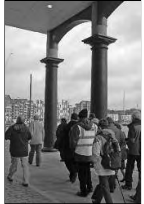
Delegates on the Ipswich waterfront at Common Quay. The cast iron columns have been re-used to support an entirely new structure, and the waterfront development can be seen in the background Photo: Lynne Walker
