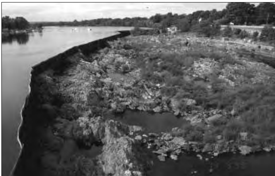
The 1093 ft long dam across the Merrimack River
