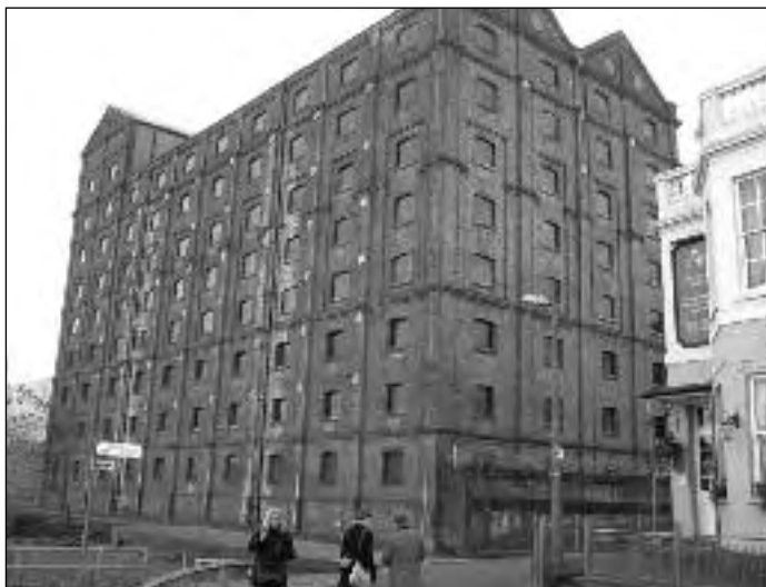
Mortlake multi-storey malthouse
