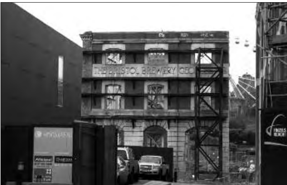
A brewery building undergoing serious redevelopment, known to some as 'façadism', seen during the Bristol day school Photo: Peter Stanier
