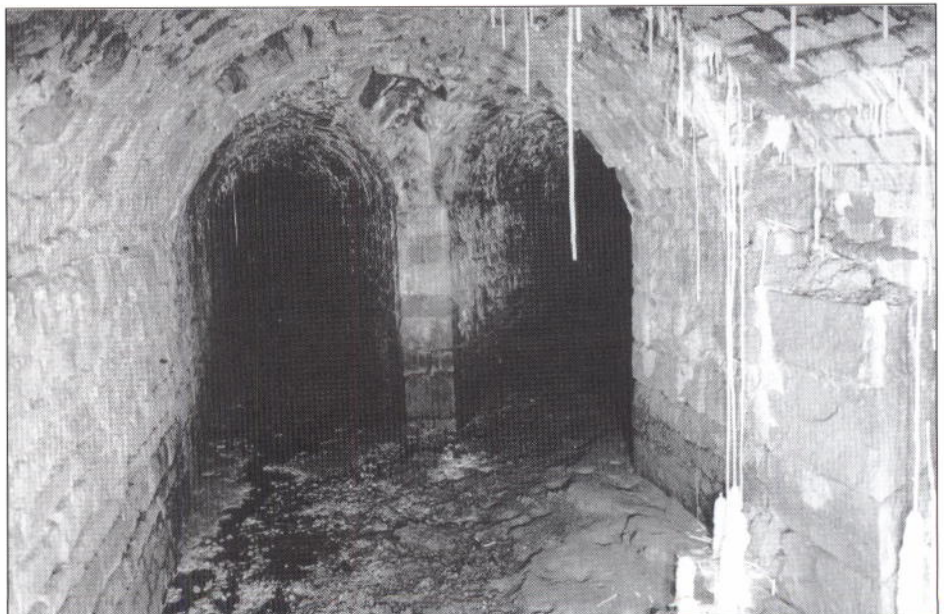
Tail races meeting to form the main culvert
