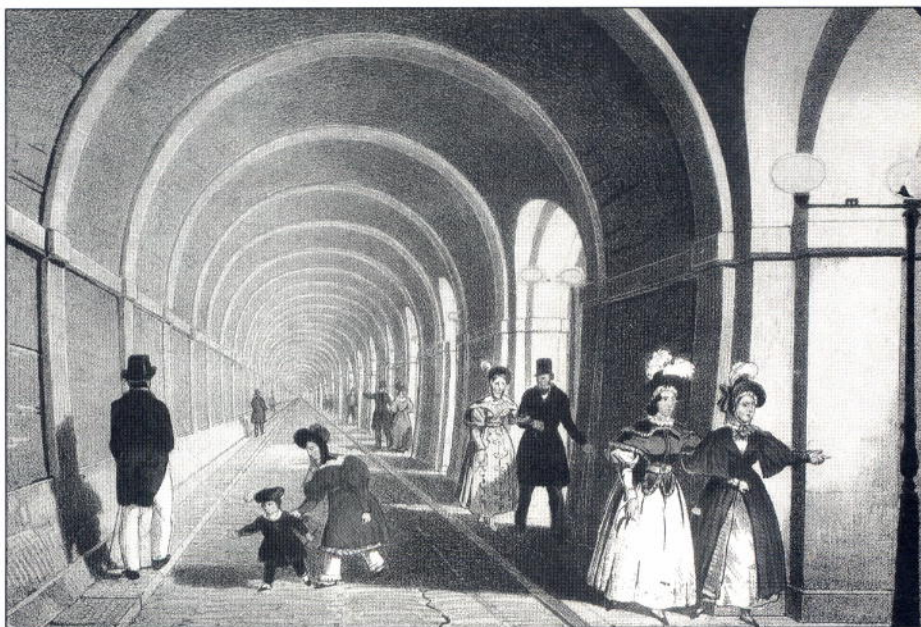
The remarkable Thames Tunnel, as seen by sightseeing visitors in the 1830s, before completion
