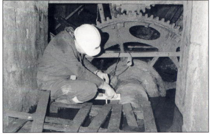
The author measuring the waterwheel, a view showing the difficult conditions encountered by the survey team Photo: M.R.I.A.S.
