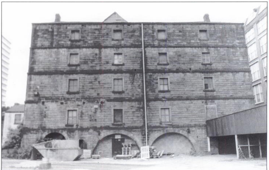
East elevation of the 1806 warehouse, showing former canal entrance
