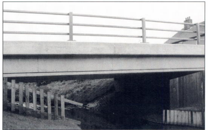
Banningham Bridge, as rebuilt in 1994-5. West elevation
