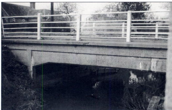
Banningham Bridge was built a year after the great 1912 flood in Norfolk. It was one of nine bridges built to a standard design. East elevation, TG231295
