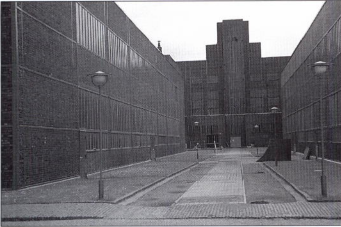
The former boilerhouse at Zollverein XII Colliery, being converted by Sir Norman Foster to the North-Rhine Westphalia Design Centre. Photo: Peter Wakelin
