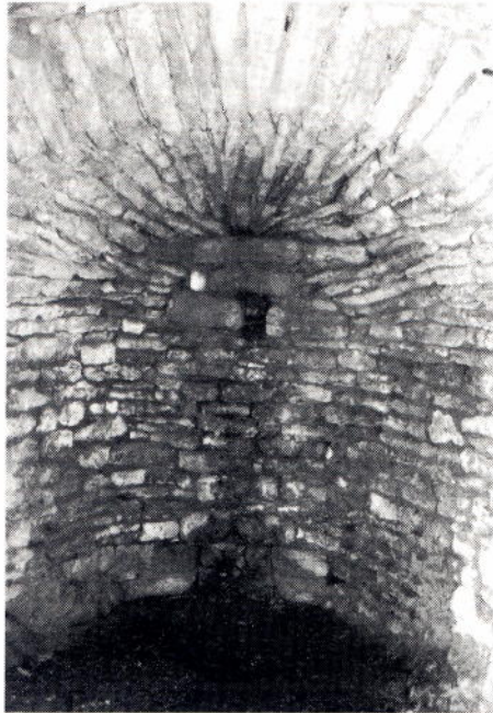
above left: Limekiln with round draw arch in stone (type A) at Longburton, North Dorset above right: Limekiln with pointed draw arch (type C) at Loders, West Dorset below: Limekiln with round brick draw arch (type B) at Woolland, North Dorset
