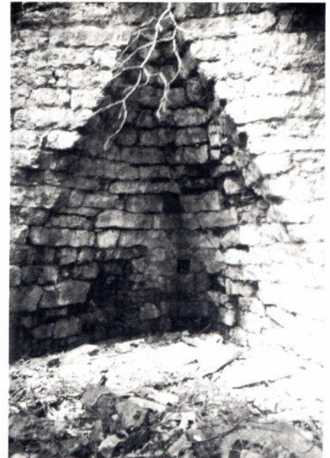
above left: Limekiln with round draw arch in stone (type A) at Longburton, North Dorset above right: Limekiln with pointed draw arch (type C) at Loders, West Dorset below: Limekiln with round brick draw arch (type B) at Woolland, North Dorset
