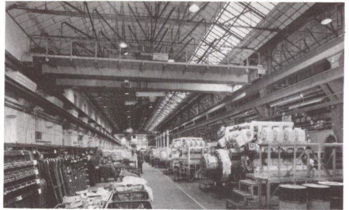
Derby Railway Works: engine assembly in the erecting shop
