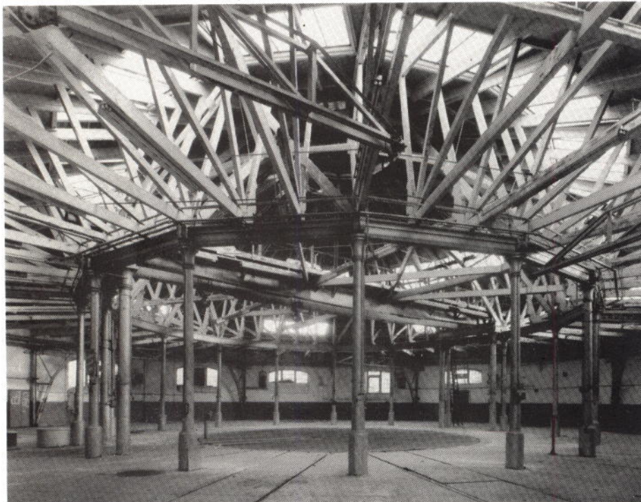
Derby Railway Works: the interior of the Roundhouse
