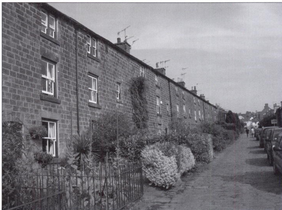
Long Row in Strutt's village at Belper, with terrace of stone houses dating from 1792-3
