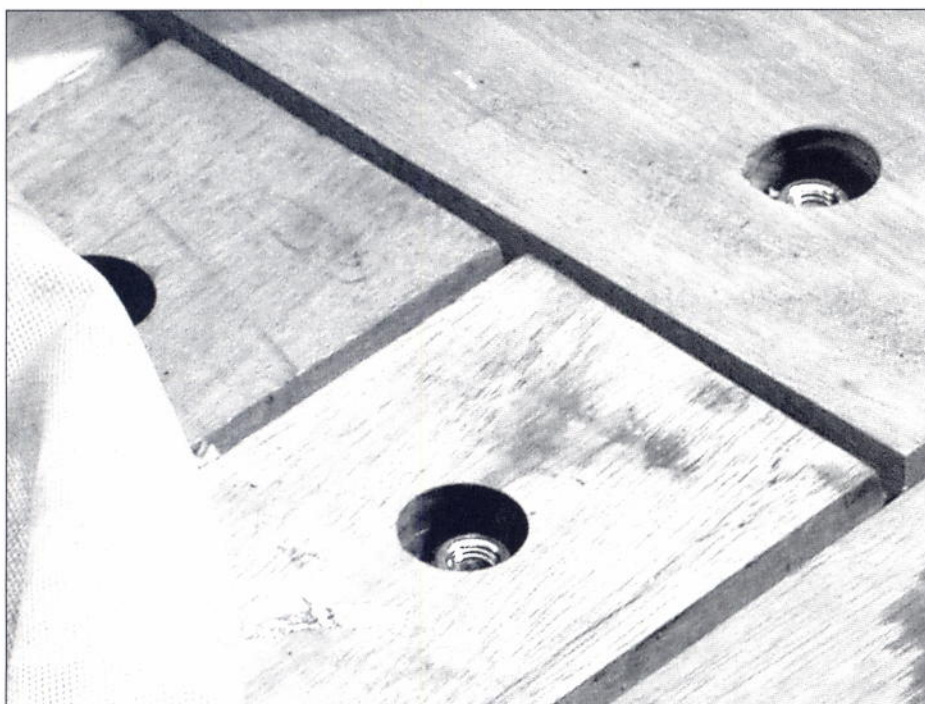
New deck planking
