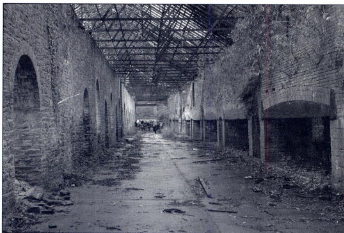
The impressive length of the derelict Treforest tinplate works
