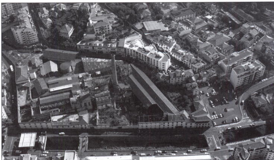
Aerial view of the Hinton Sugar Mill, Madeira
