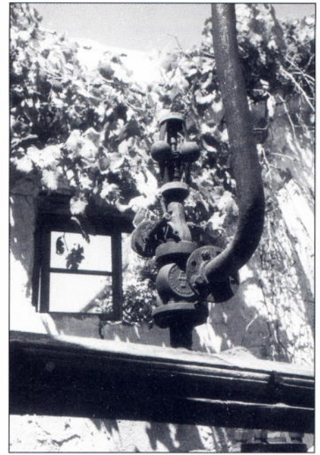
Pickering Combination steam governor assembly supplied for the Averly horizontal steam engine, seen inside the collapsed engine house Photo: Paul Vigor
