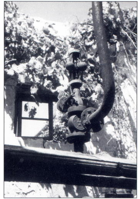
Pickering Combination steam governor assembly supplied for the Averly horizontal steam engine, seen inside the collapsed engine house Photo: Paul Vigor
