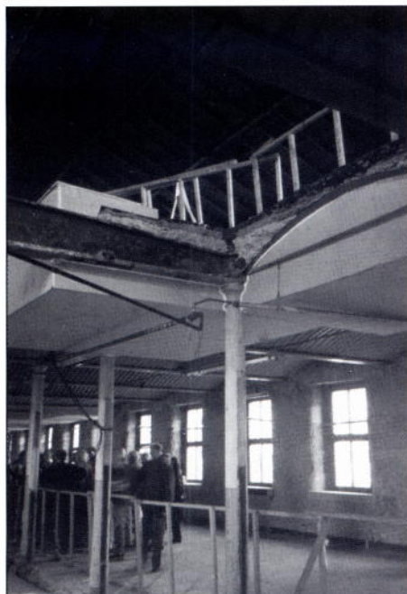
A detail of the fireproof floor and ceiling supported by corrugated iron arches in the Great Eastern Hotel (1840s cotton mill), Glasgow
