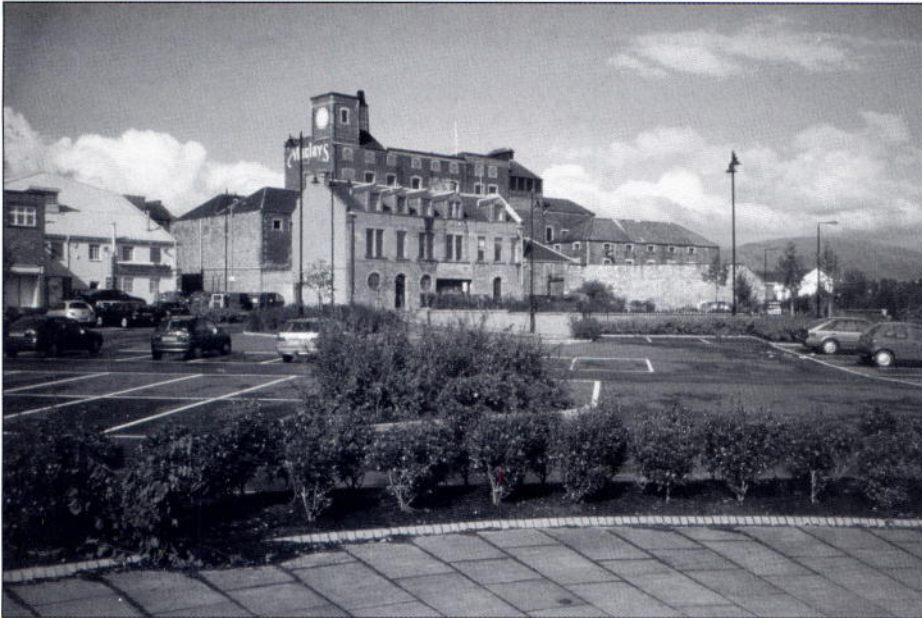
Maclay's Thistle Brewery at Alloa, closed but intact and awaiting redevelopment
