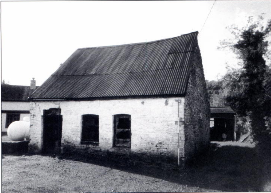
The roadside smithy, viewed from the north-east, beneath a corrugated roof
