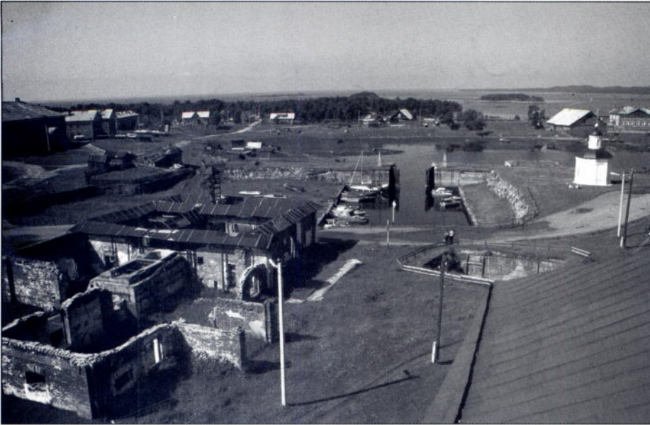
The hydro-electric station remains with the dry dock beyond, seen from the monastery fortifications. The roof on the left is the grain store Photo: Mike Clarke
