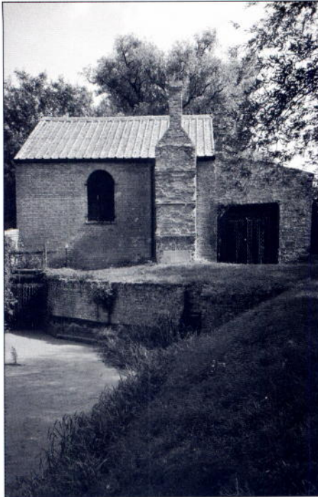
West Fen engine house
