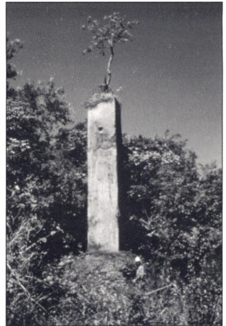
Blast furnace of the Guazucarán complex Photo: Pastor Gómez
