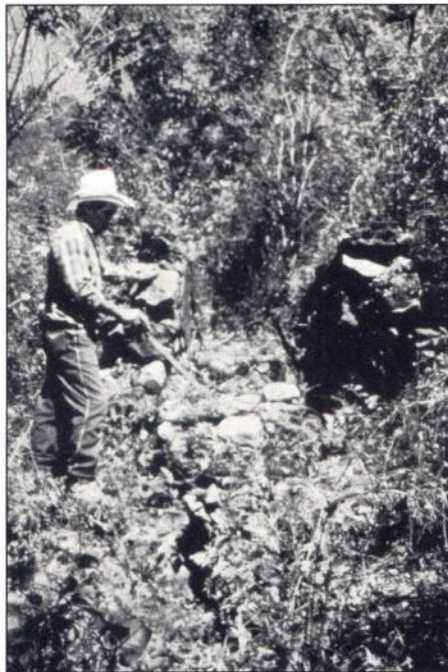
Section of the water canal, built with rubblework, at Guazucarán Photo: Pastor Gómez
