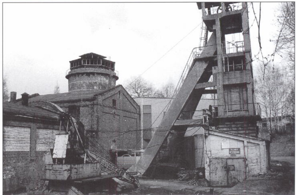
Circular masonry ventilating tower or évasée of 1898 and later reinforced concrete shaft, Debiensko colliery
