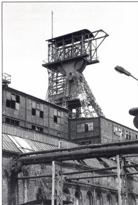
One of only three remaining headstocks with pyramidal backstays, Petrowski colliery, 1902
