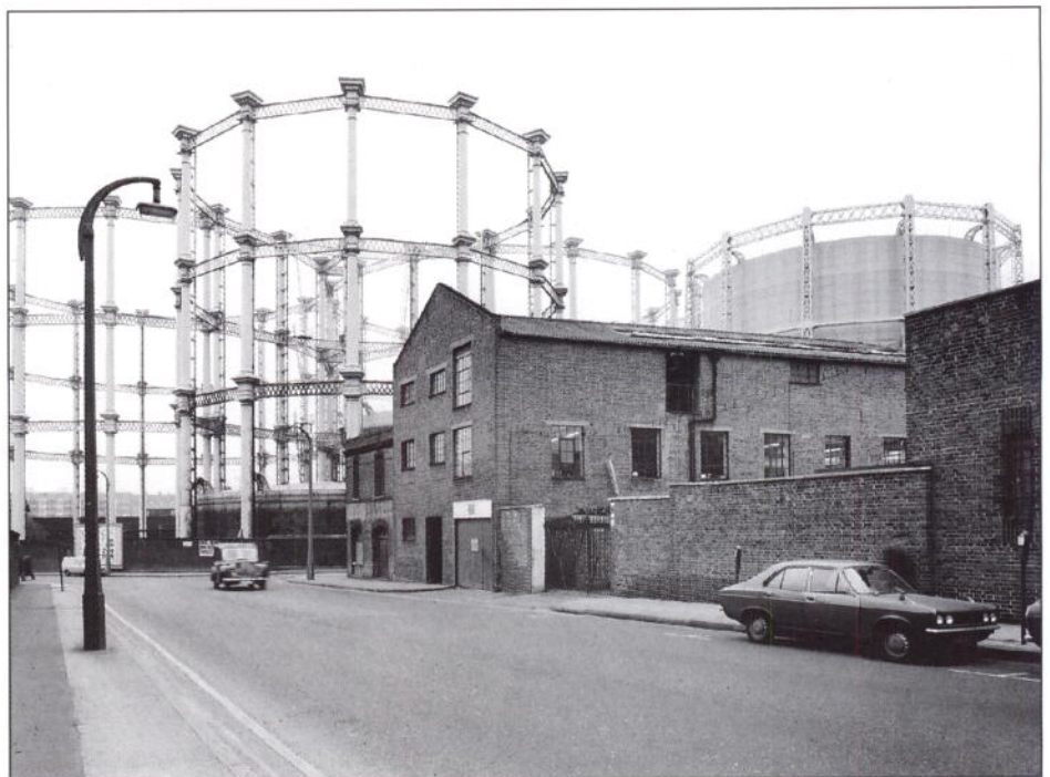
The famous linked triplet of gasholders, nos. 10, 11 and 12, as rebuilt by John Clark, 1879-80. All listed grade II, they are to be re-erected to make way for the Channel Tunnel Rail Link
