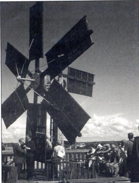
Windmill once used for pumping brine to the top of a tower Photo: M. Palmer
