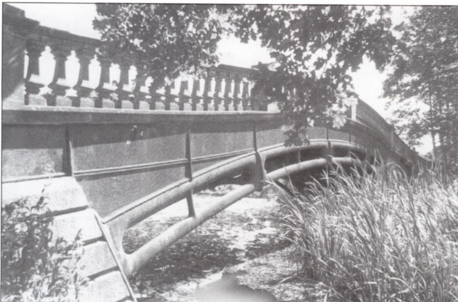
Detail of iron arch, showing the stone balustrade above
