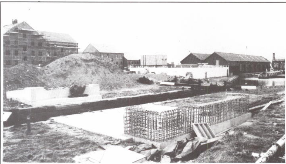
Redevelopment around Ellesmere Port. A new access bridge is being built across the Barge Lock to the Lower Basin for the proposed hotel on the basin's centre island: the bridge's structure and design has been the subject of some debate. The new buildings behind are part of the 'Telford Quays' development.
