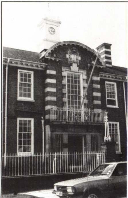
Marconi's New Street Works, Chelmsford Photo: L F Roberts
