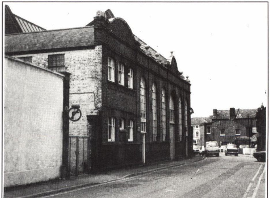
The remaining portion of Crompton's first works, Anchor Street, Chelmsford
