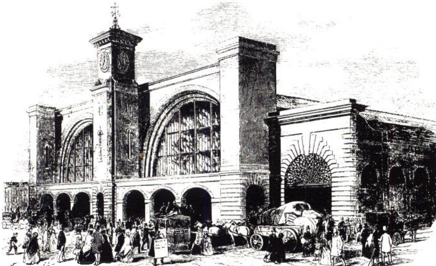
King's Cross station looking north, about 1853.
