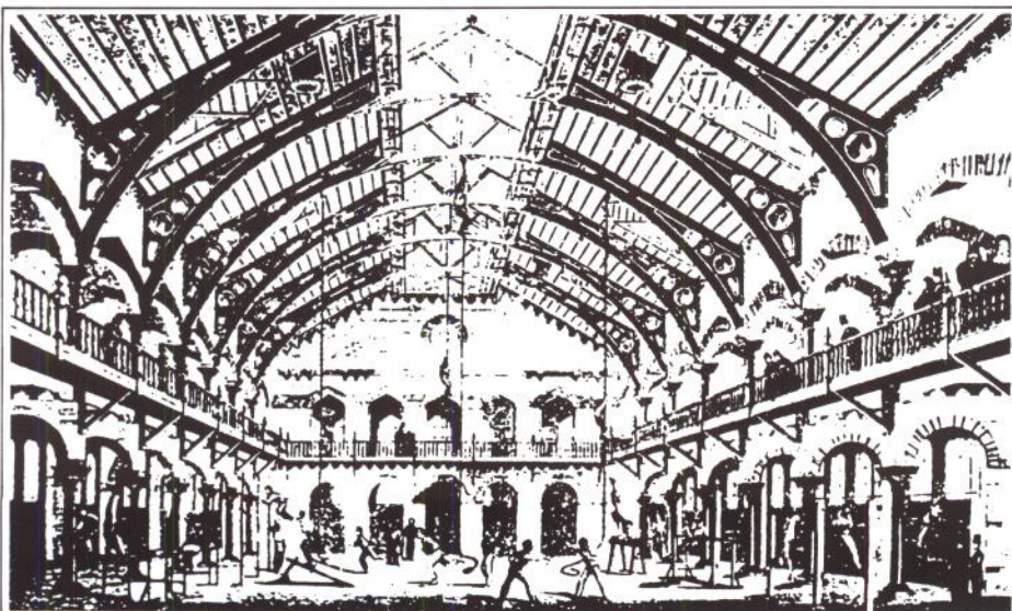
Interior of the German Gymnasium. The roof is supported by laminated timber arches.
