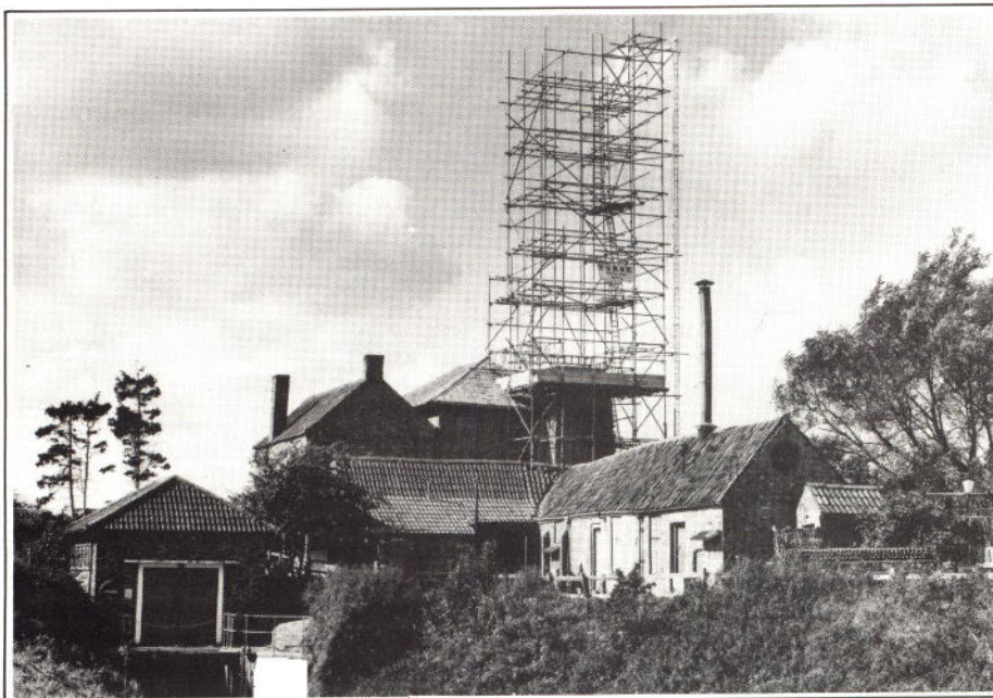
Hole in the sky: the main stack at Westonzoyland after dismantling and shortly before re-erection. Photo: Ian Watts
