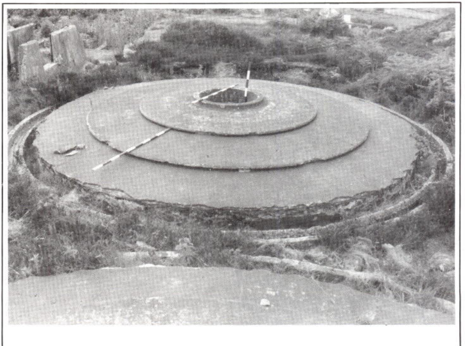
3. Stepped buddle, Brea Adit tin-streaming site, Cornwall, early 20th century.
