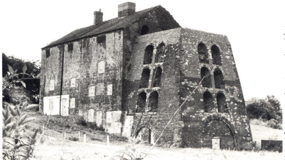
Moira furnace prior to restoration
