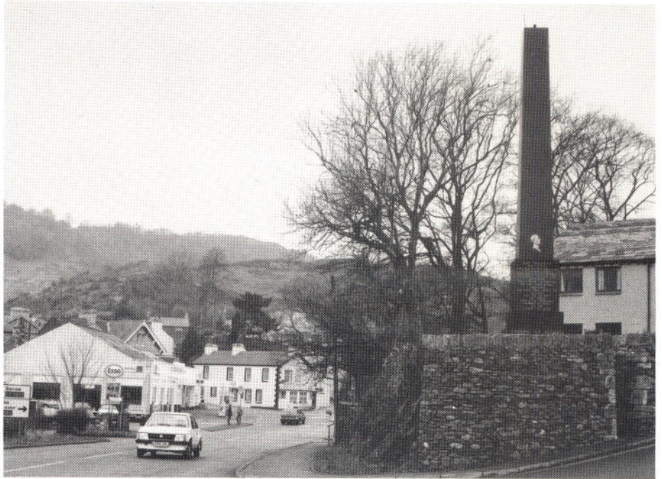
The recently-restored John Wilkinson Monument at Lindale in Cumbria.
