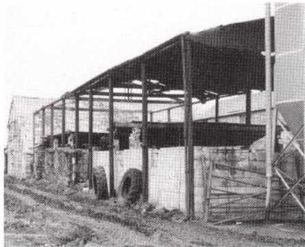
A cow shed at Wilson House Farm is supported by cast iron pipes made for the Paris Waterworks. They must have been surplus to requirements, as the Paris contract was completed successfully.
