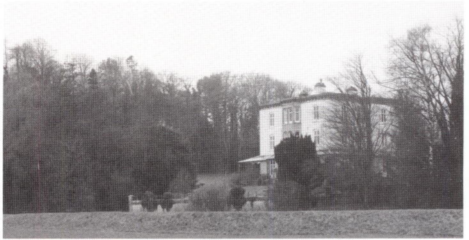
Castle Head, Wilkinson's home from about 1779 onwards. The monument originally stood in the trees to the left of the house before being taken down by the Mucklow family in the 19th century.
