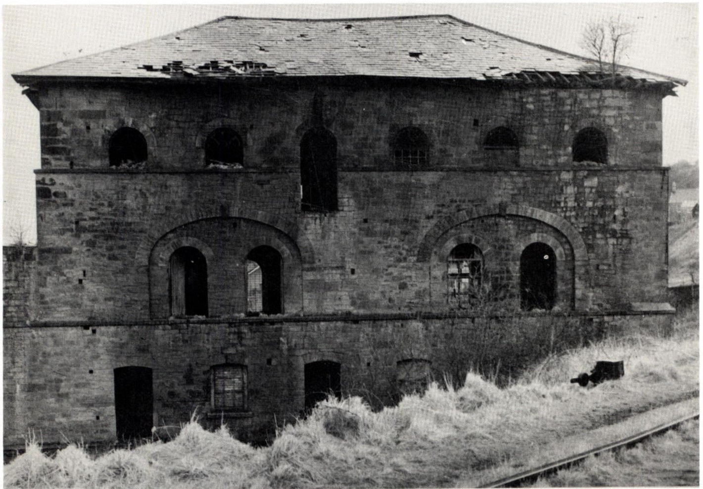
The great engine house at Maesteg
