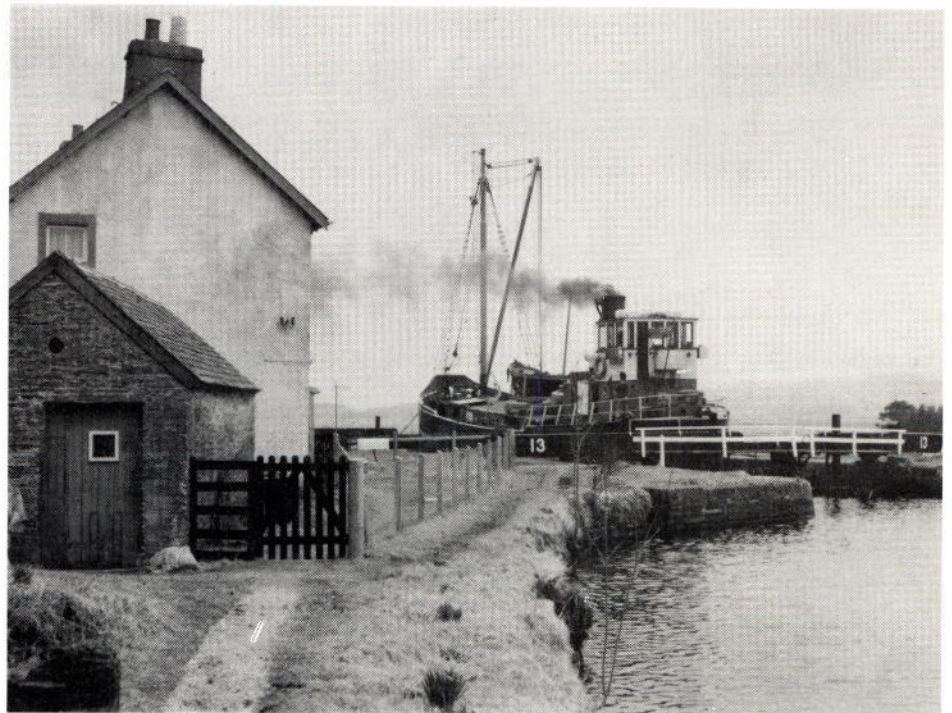
VIC 32 at Dunardry Locks on the Crinan Canal
